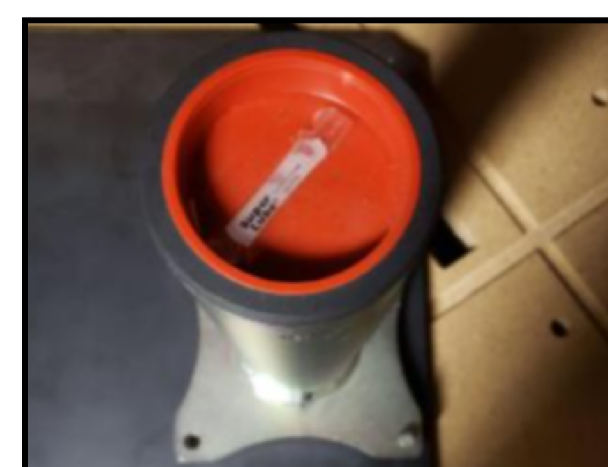
Fabrication of Crane Base
