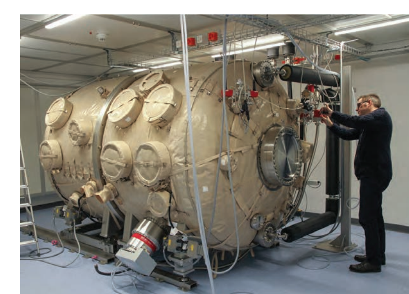
Full System Validation On Site at ASML
