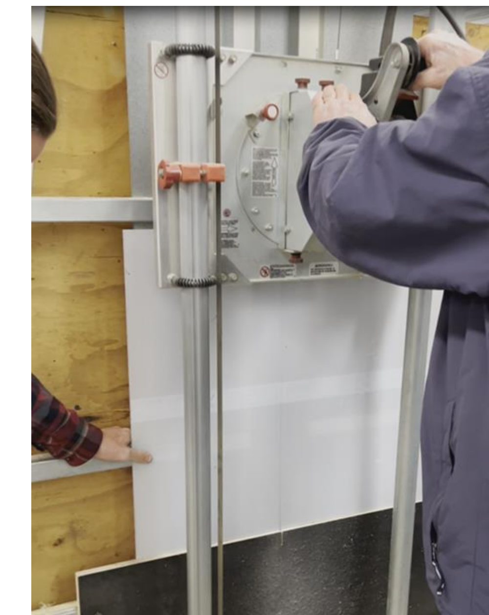
Figure 9: Cutting Polycarbonate Panels to Size with Wall Saw
